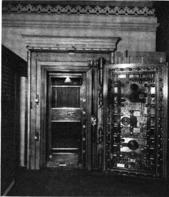
Entrance to the Safe Deposit Vault
